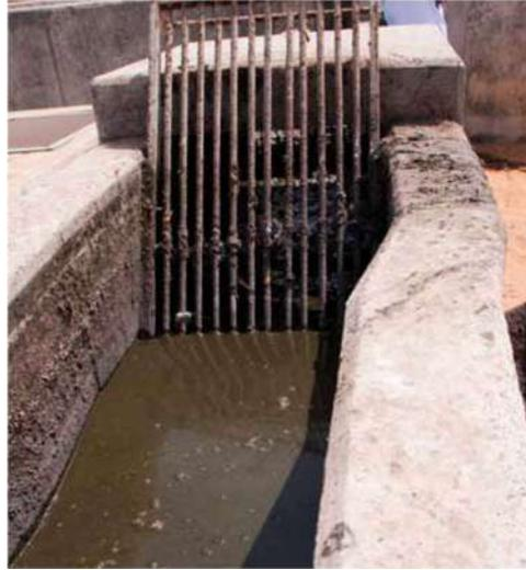
Fig 2: A typical manual screen channel in the septage plant. (Source: Linda Strande)
